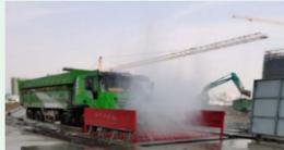
A car washing pool was set up to achieve one-time water supply, which was then recycled after three-stage sedimentation. A dedicated person was responsible for controlling dust on the construction site, using effective measures such as sprinkling water, enclosures, and covering to minimize dust emissions.
